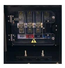
Main bus connection studs enclosed behind a lockable access door for easy access and operator safety.
